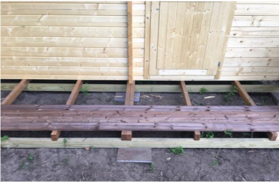
42. Install the porch (terrace) boards (TB1-1) starting at the front and working your way back toward the sauna. Place the narrow porch board (TB1-2) at the front and between the front porch rails. Nail the porch boards to the foundation stringers. NOTE: If the porch boards do not reach far enough to cover the left and right stringers, you can nail a support piece into the stringers and nail into it.
