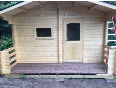
43. View of completed porch.
