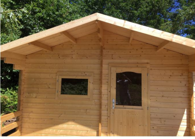
41. View of sauna after fascia boards attached.
